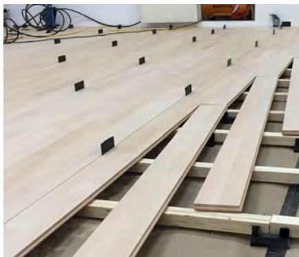
The boards are tongue and groove on all edges, and fit together. A modern court like this is secret-nailed in the tongue at an angle of 45 degrees which allows the groove of the next board to sit snugly against its neighbour. Nails are not then visible on the surface, as you see in older courts. The boards in this Junckers system have a header joint where the end of the boards sits on a batten; this supports the end. The credit-card size black spacers are for a 2mm ‘washer gap’ to allow for expansion so that the floor does not buckle. This closes over time
